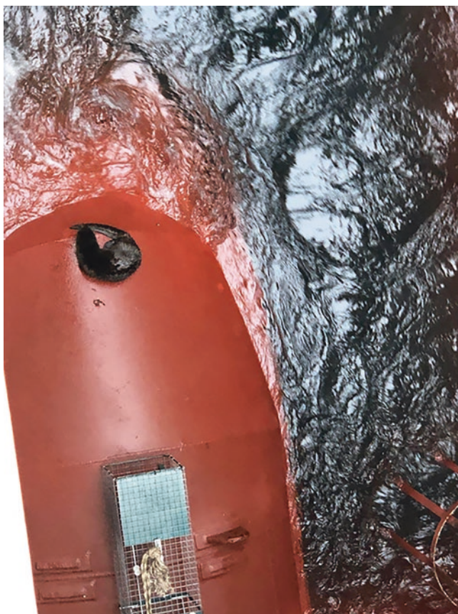
Fig. 7.3 Marine otter trapped in the intake well of the cooling process at AES GENER company. (Source: Servicio de Pesca y Acuicultura Región de Valparaíso, Chile)
