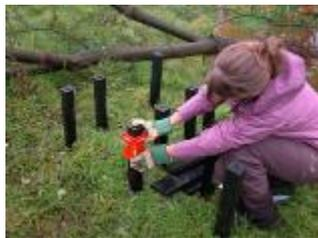
3) Fit the inner walls (there is not room to operate the drills with the outer walls in place). It does not matter whether the tongue or the groove in the plank is uppermost as long as all the walls are the
