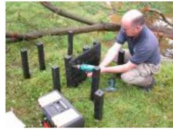
Drill and screw the top row first, locating the planks 10mm down from the top of the posts. This is to make a gap which will create a little airflow, reducing condensation forming inside the holt. Slide the lower planks onto the upper ones locking them using the tongue & groove slots and screw them in. Any gaps at the bottom can now be made up with soil. **IT IS IMPORTANT TO FOLLOW THE PLAN EXACTLY.** If the plan says that a corner lines up like this:
