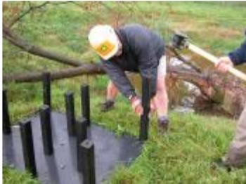
2) Hammer in the posts, using the holes in the template, to a height of 43cm (17"), remove the template and level the posts accurately using the spirit level and corner post level.
